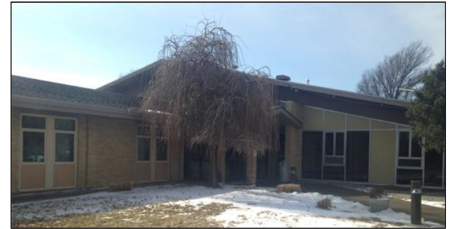
Olathe Mental Health (OMH) 1125 W. Spruce Street, Constructed in 1966
